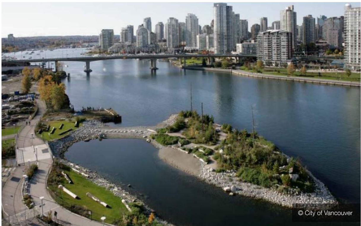
The constructed Habitat Island.
